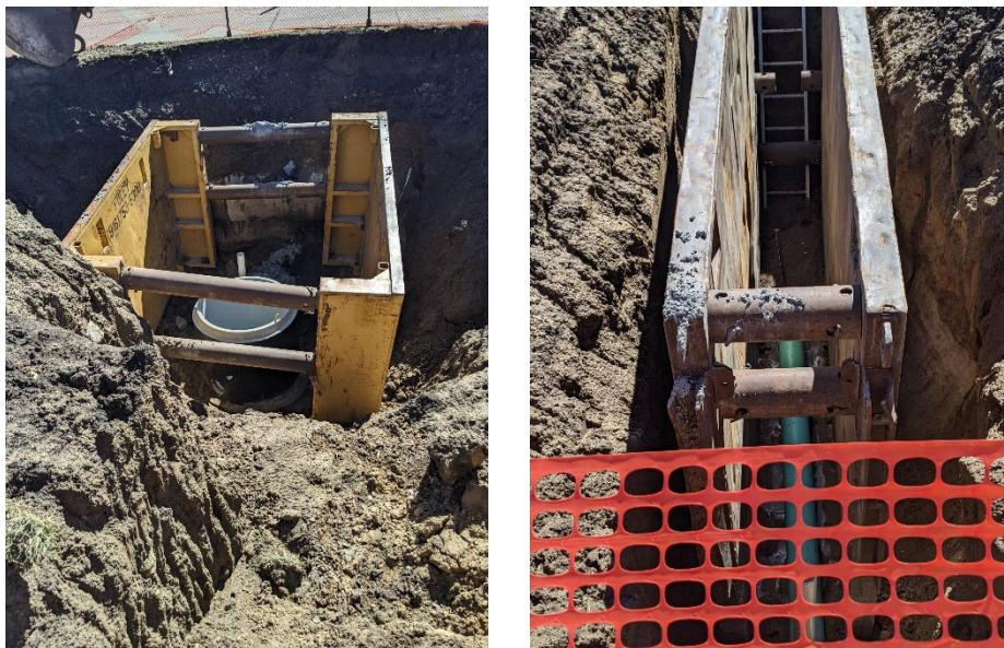
Here is a couple of shots from the Dexter & Ford intersection area where sanitary sewer is being brought across Ford Street. The left shot shows a new manhole being installed as part of the strategy to re-route this around some gas equipment there on this corner. The other shot of some of the sanitary sewer being install on the south side of Ford Street.
